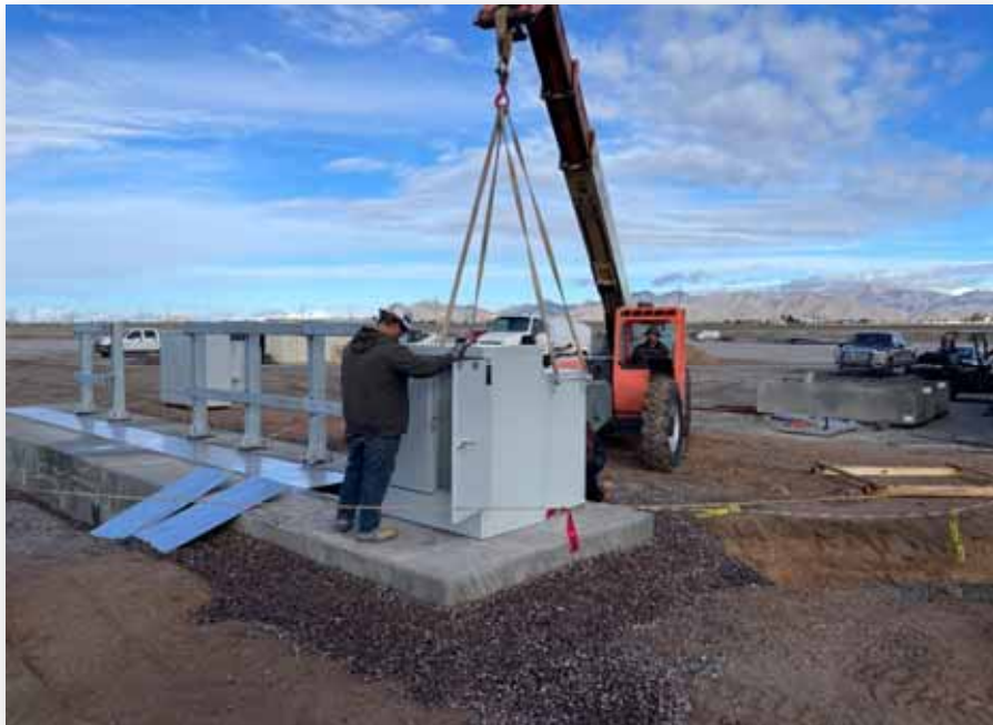
Figure 6. WAPA Maintenance personnel setting transformer KY2B
