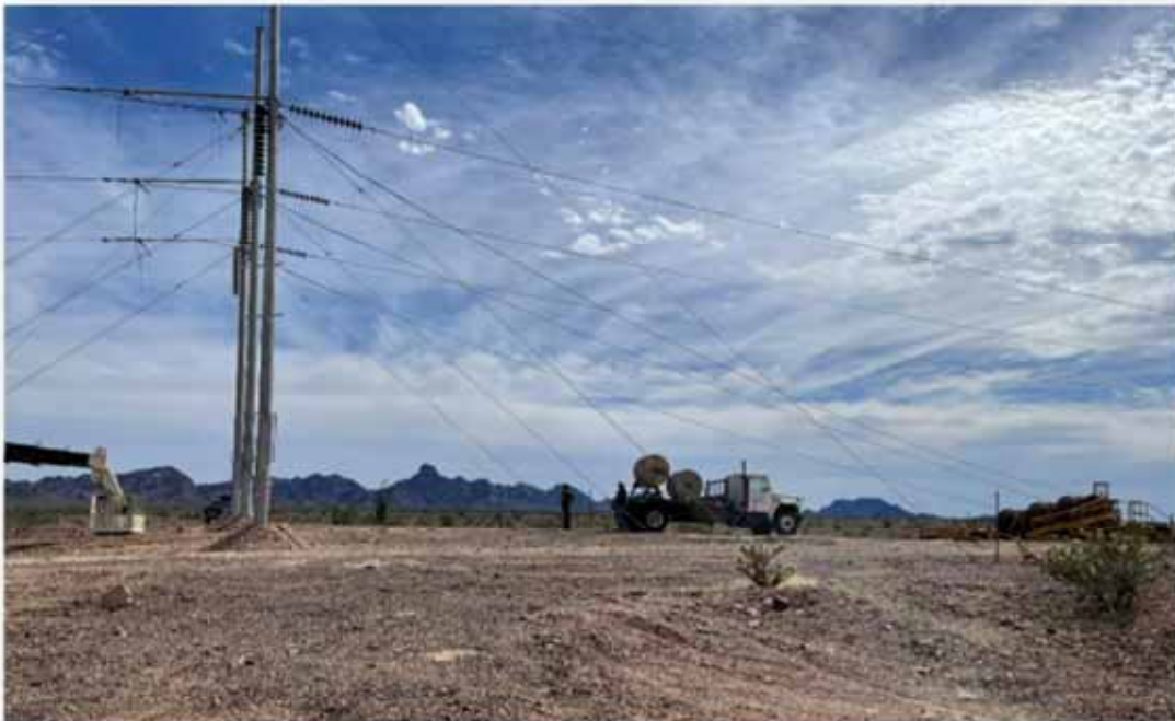
Figure 4. Crew setting up to pull in the new OGW at BSE-KOF 82/10 structure.
