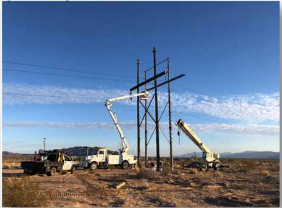
Figure 3. Crew erecting new BSE-KOF 103/6 structure.
