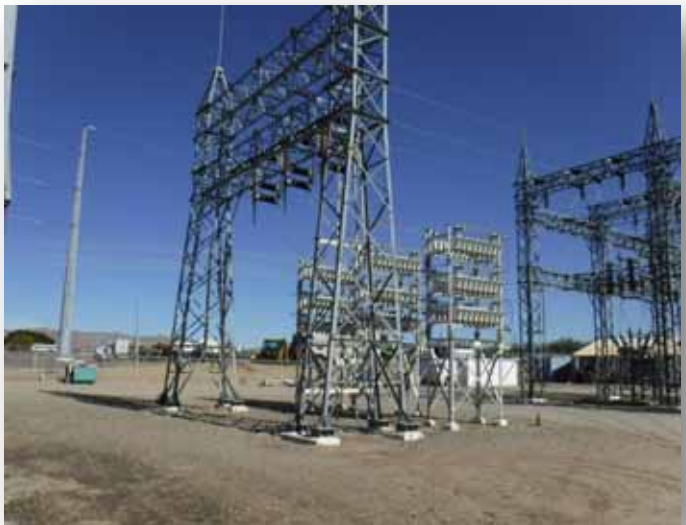
Figure 2. Crew erecting new BSE-KOF 103/6 structure.
