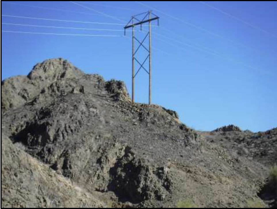
North view of Structure 2/6
