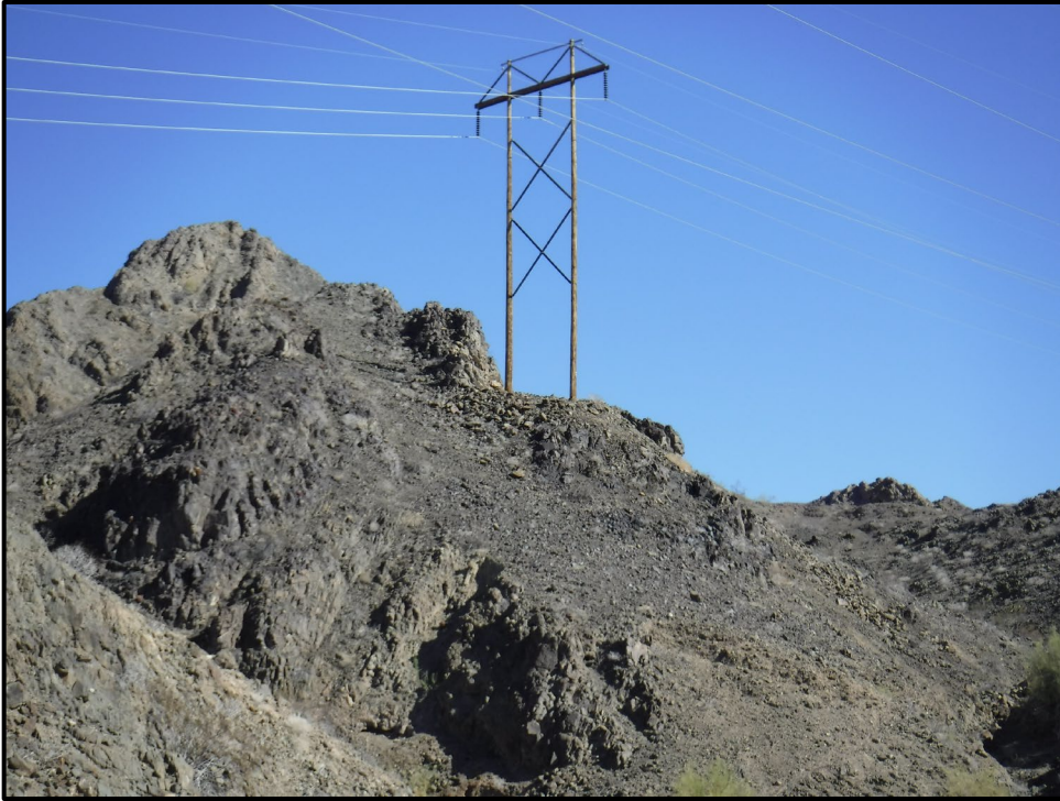
North view of Structure 2/6
