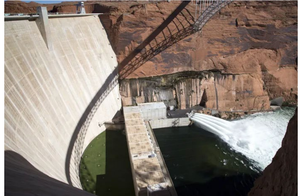
Bypass at Glen Canyon Dam
