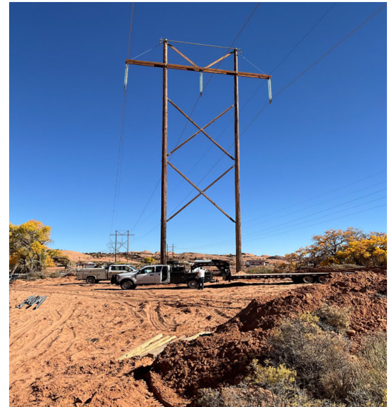
Temporary Fix: October 2025, we removed failing lattice structure and installed 2 H-Frames for stabilization
