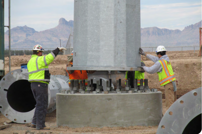
Construction crews secure the next section of the Saguaro line structure that is part of the Electrical District No. 5 substation upgrade. WAPA file photo
