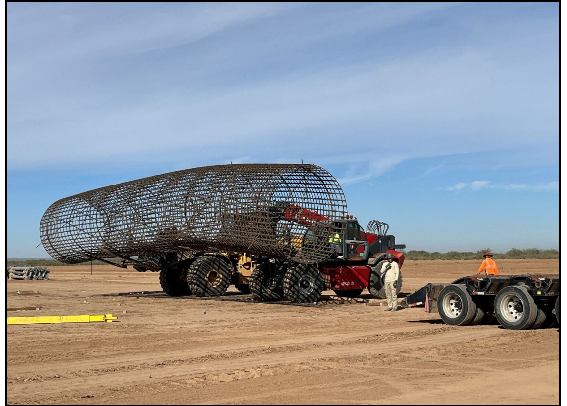
Anchor Bolt Cage
