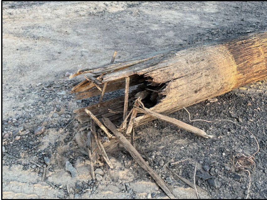
Severe pole rot visible after removal
