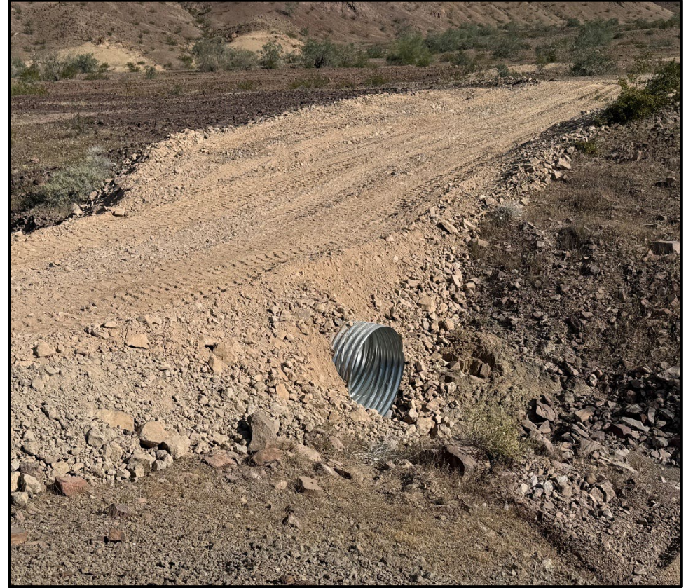
Culvert replacement on mile 20
