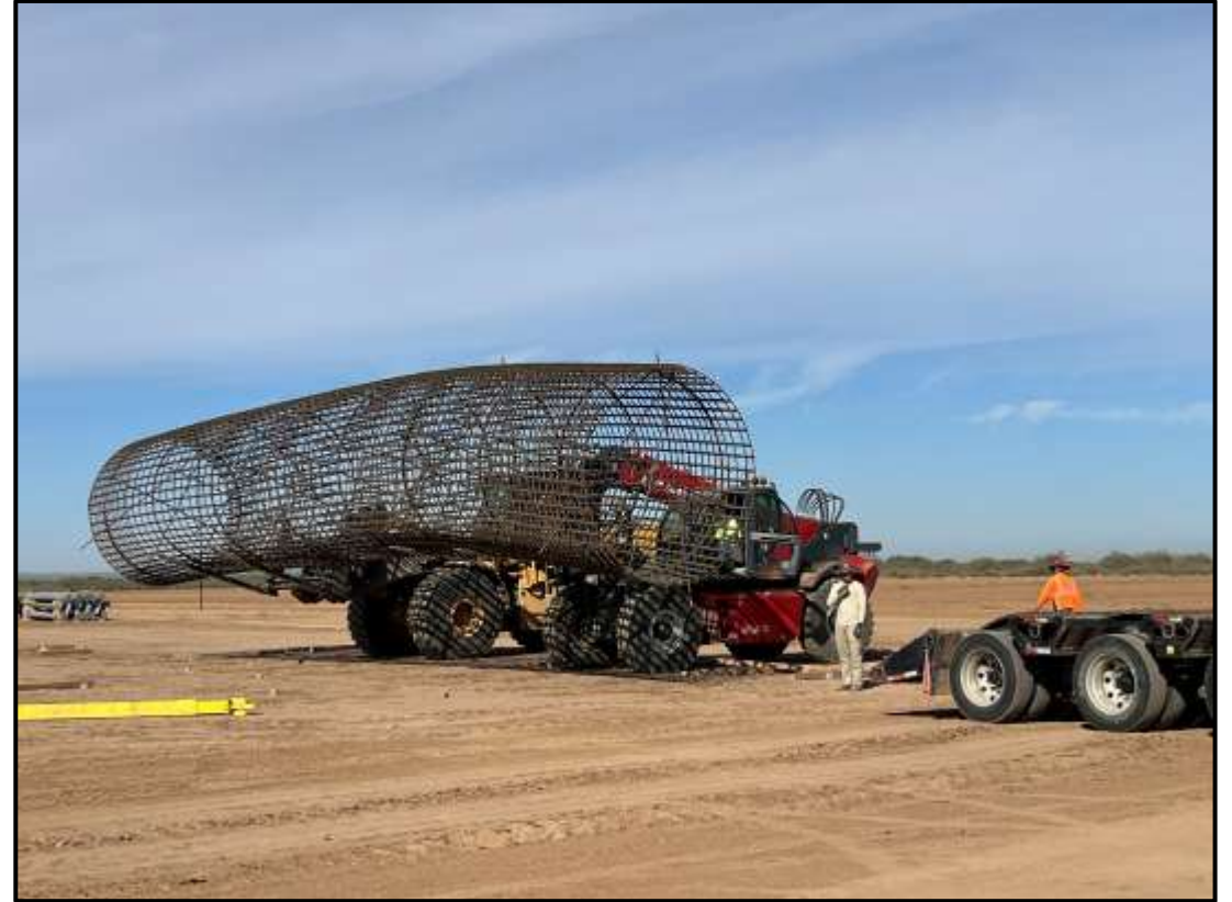
Anchor Bolt Cage
