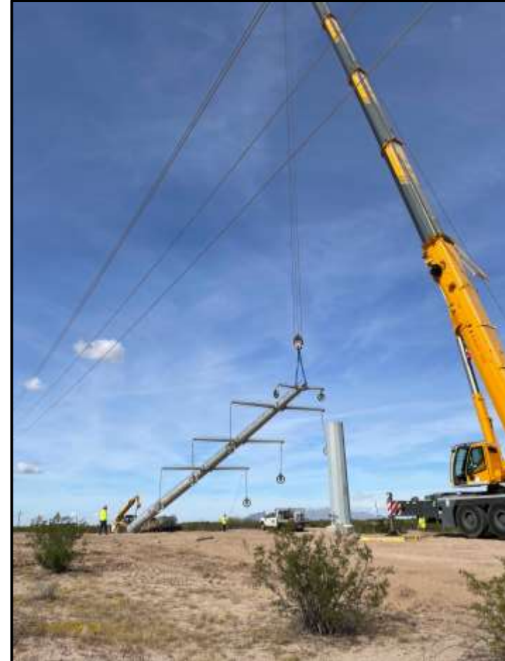
Steel monopole erection
