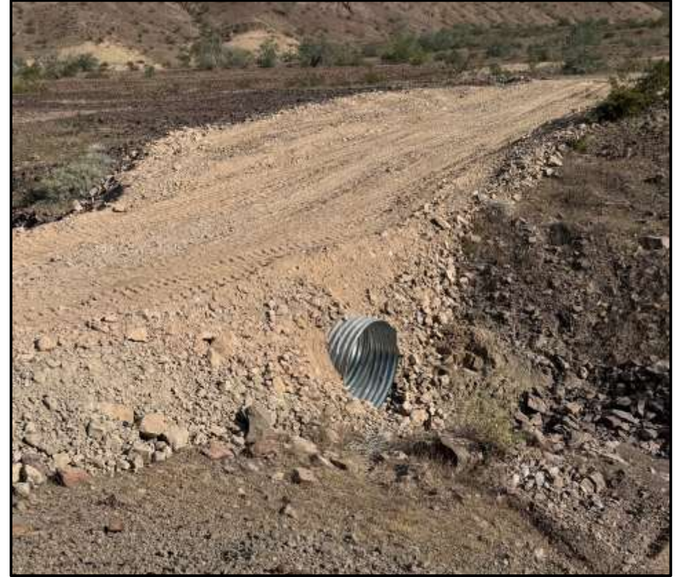
Culvert replacement on mile 20
