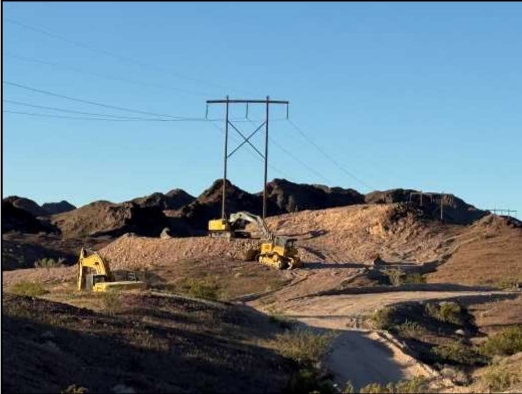
Sitework equipment on BLY-KNB right-of-way
