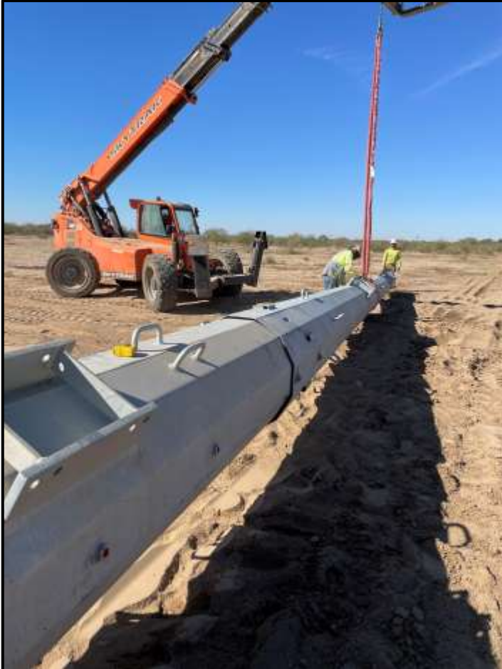
Steel monopole assembly
