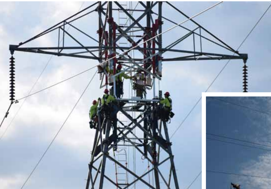
A contracted crew uses new technology to raise a steel lattice structure in South Dakota, Aug. 12, to ensure compliance with ground clearance regulations. This is one of 37 towers Upper Great Plains will raise this summer and fall. (Photo provided by Cody Kinsley)
