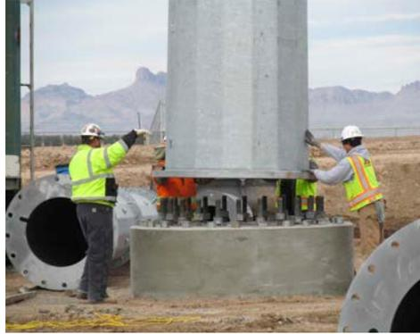
Construction crews secure the next section of the Saguaro line structure that is part of the ED5 substation upgrade. *Photo from Ralph McCracken, Western Area Power Administration*
