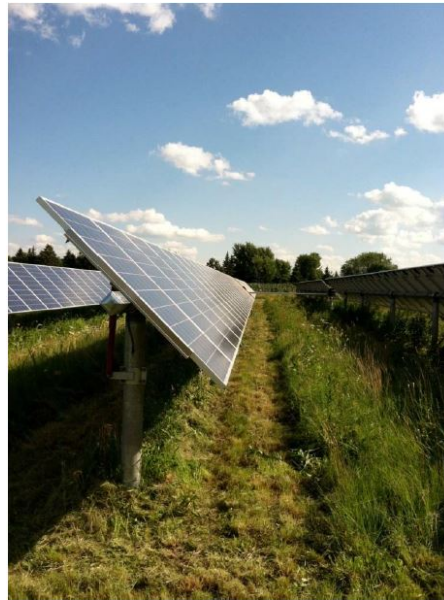
Image 1 Tracking Rack System and Solar Panels at 45-Degree Angle
