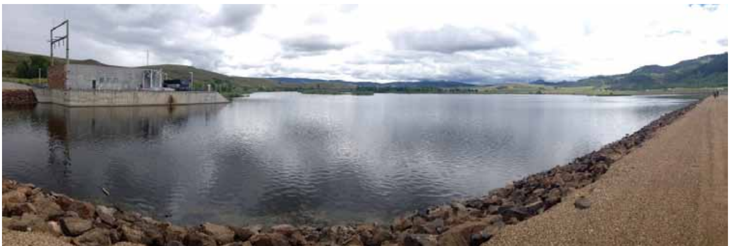
A panoramic view of Windy Gap Pumping Plant and Windy Gap Reservoir. (Staff photo)
