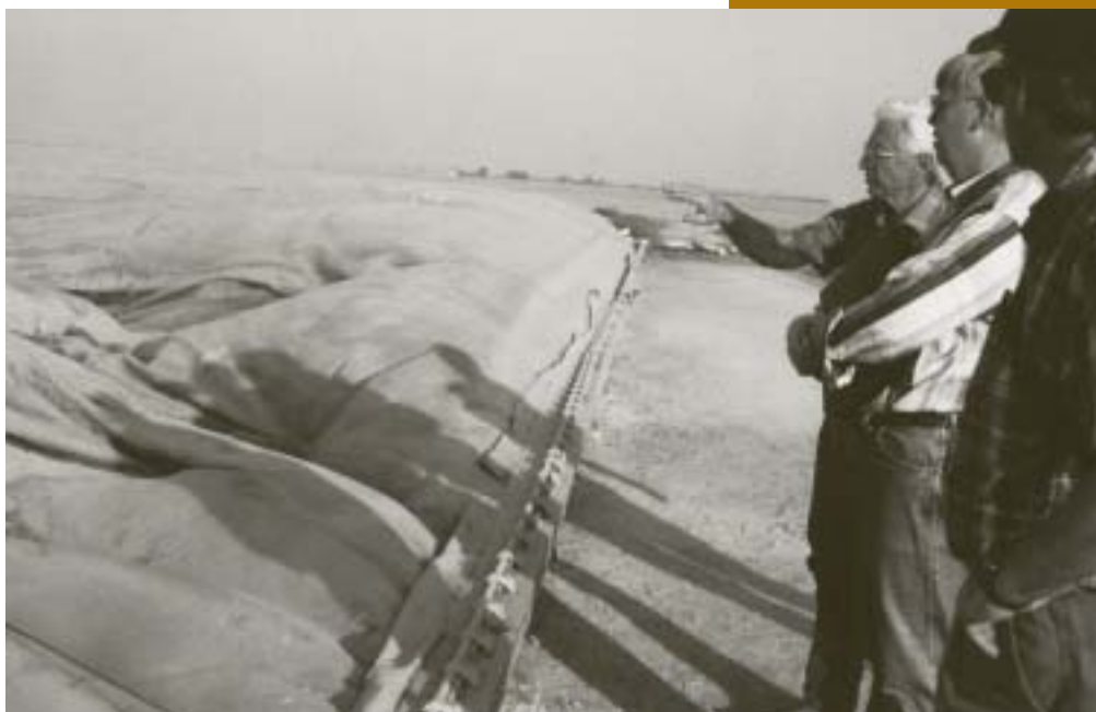
The Western Regional Biomass Energy Program encouraged the use of technologies such as anaerobic digestion, which breaks down animal wastes to produce biogas. The biogas powers a generator to produce electricity. A cover on a manure lagoon traps the biogas.
