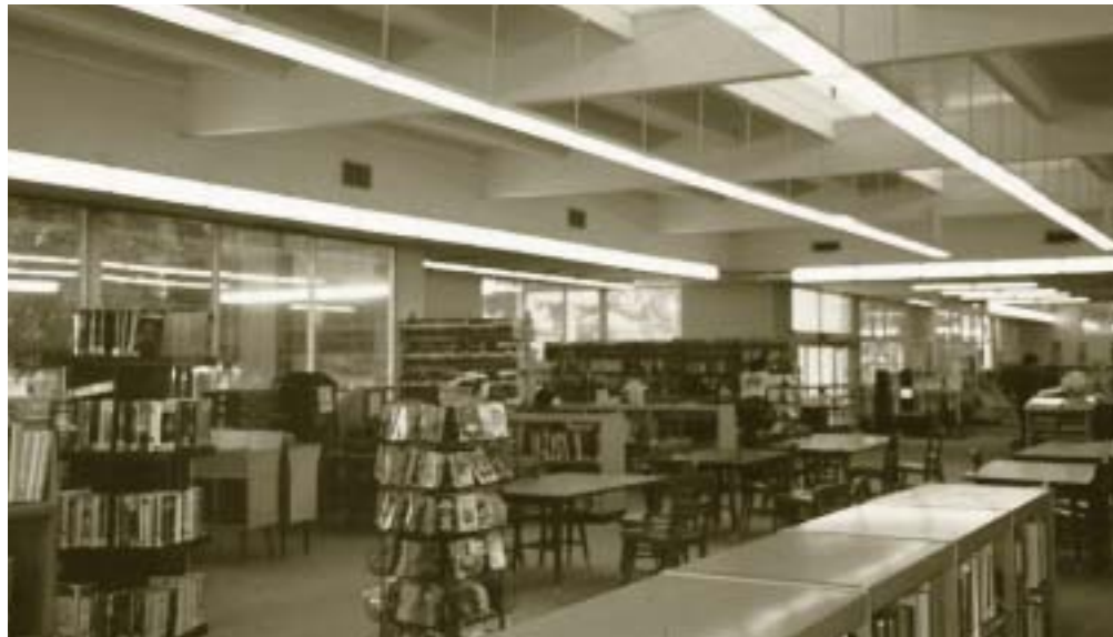
Western's customers encouraged energy savings through efficient lighting installations like this one at the Azusa Public Library in 1994.
